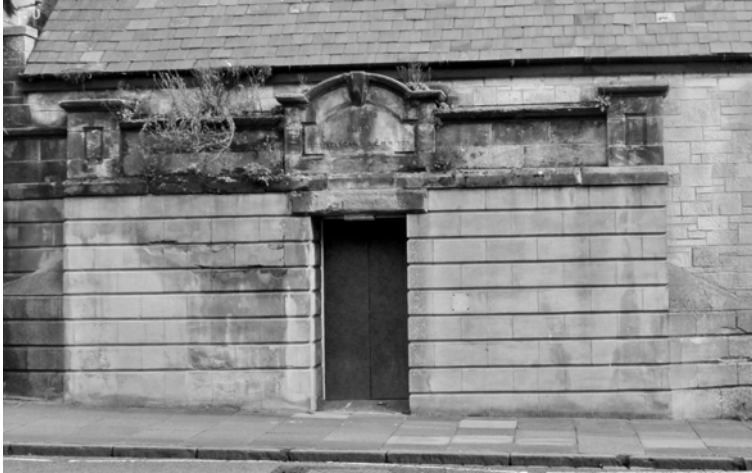
Conduit Head building
